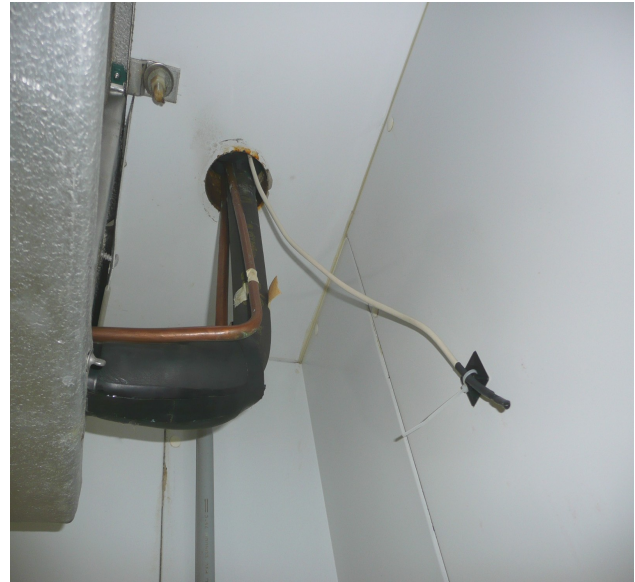
Temp sensor in cold room
